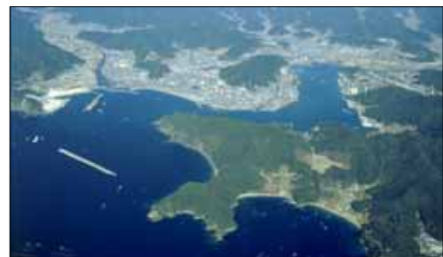
Fig.13 Tsunami breakwater in Suzaki
