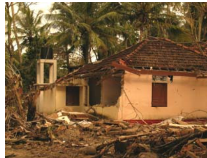
Fig. 2 - Reinforced Concrete frame with non-structural infill (Courtesy of EEFIT)
