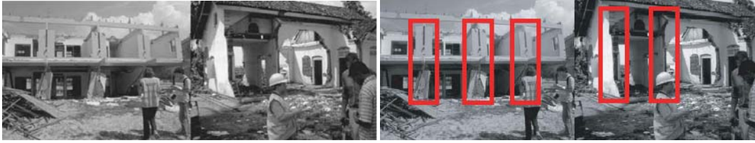
Fig. 5 - Partially collapsed structures after the 2004 Tsunami in Sri Lanka
