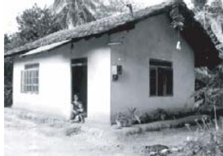
Fig. 3 – Traditional house being rebuilt in Sri Lanka
